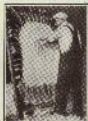
Stretching calfskins for Ludwig drum heads
